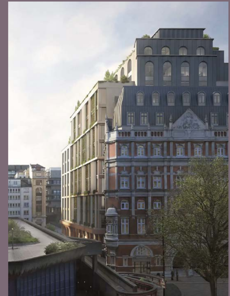
View showing the retained grade II listed facade Source: Planning Application DAS
